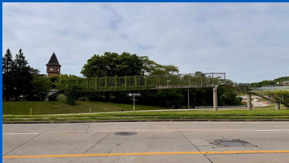
Pedestrian bridge over W. Fifth St. exit off-ramp
