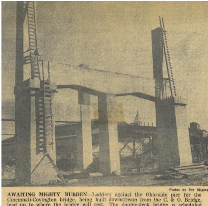
AWAITING MIGHTY BURDEN—Ladders against the Ohio-side pier for the Cincinnati-Covington bridge, being built downstream from the C. & O. Bridge, lead up to where the bridge will rest. The double-deck bridge is scheduled for completion in May 1963. Photos by Bob Stigers
