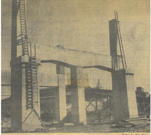
AWAITING MIGHTY BURDEN—Ladders against the Ohio-side pier for the Cincinnati-Covington bridge, being built downstream from the C. & O. Bridge, lead up to where the bridge will rest. The double-deck bridge is scheduled for completion in May 1963.
