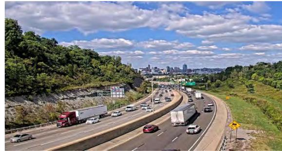
*Long, steep roadway grades can negatively affect traffic flow on interstate highways such as on southbound I-71/I-75 between Kyles Lane and MLK Jr. Boulevard in Kentucky – also known as the “Cut in the Hill” (pictured above). Truck traffic climbing the hill often moves at a much slower speed than other traffic. The substantial difference in speed between trucks and cars contributes to elevated traffic congestion and crashes.<sup>1</sup> (Photo: Traffic cam for I-71/I-75 at Cut in the Hill)*
