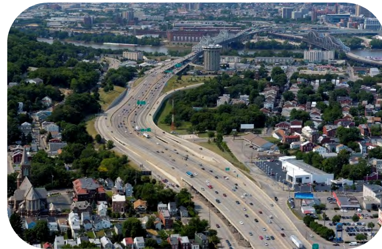
Kentucky approach to Brent Spence Bridge
