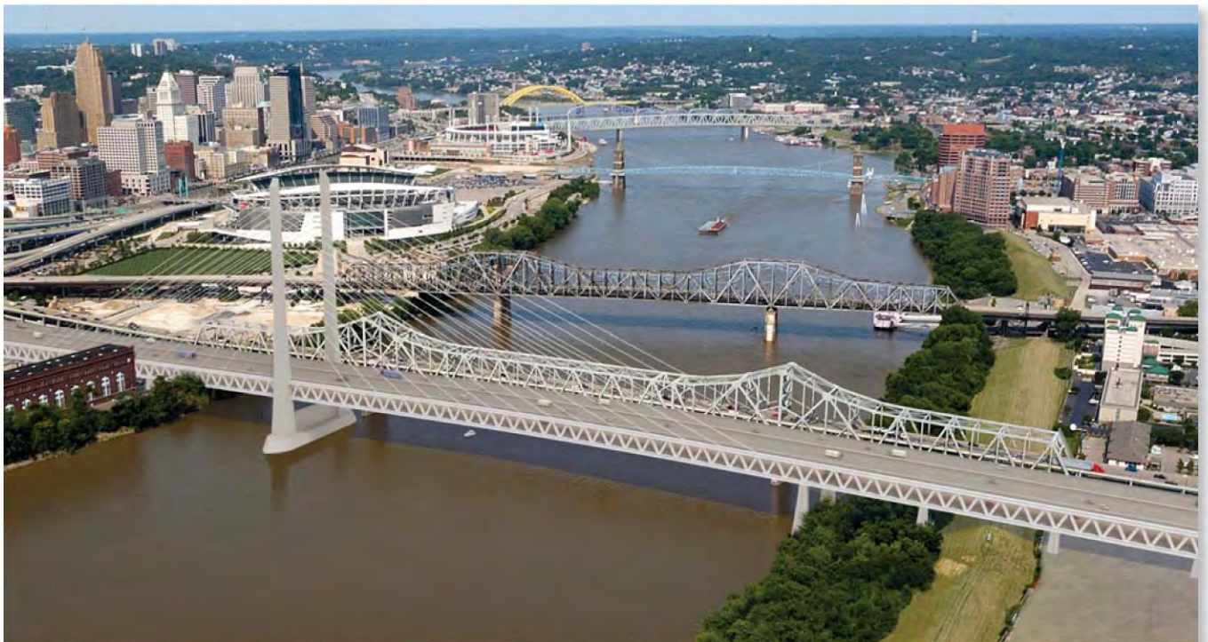
Alternative 6: One Tower Cable Stayed Bridge
