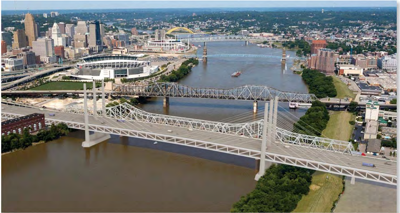
Alternative 3: Two Tower Cable Stayed Bridge
