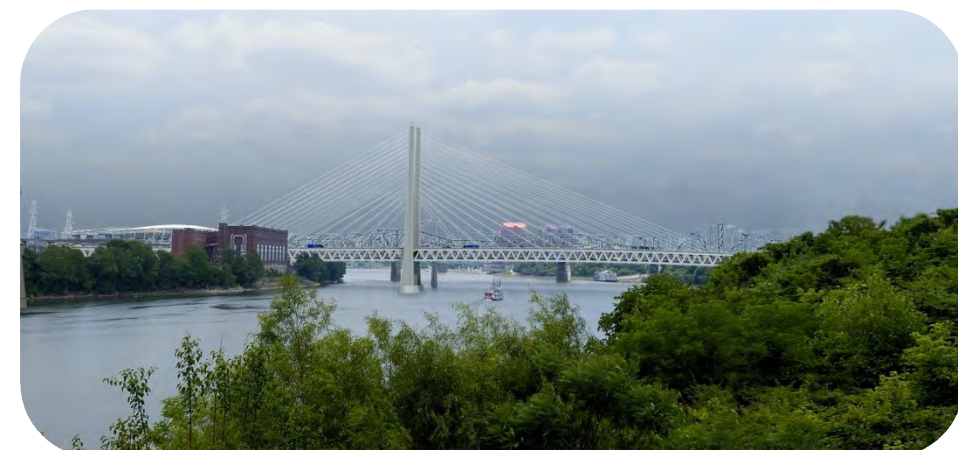
Alternative 6 – Single Tower Cable Stayed (2-Needle-Tower)
