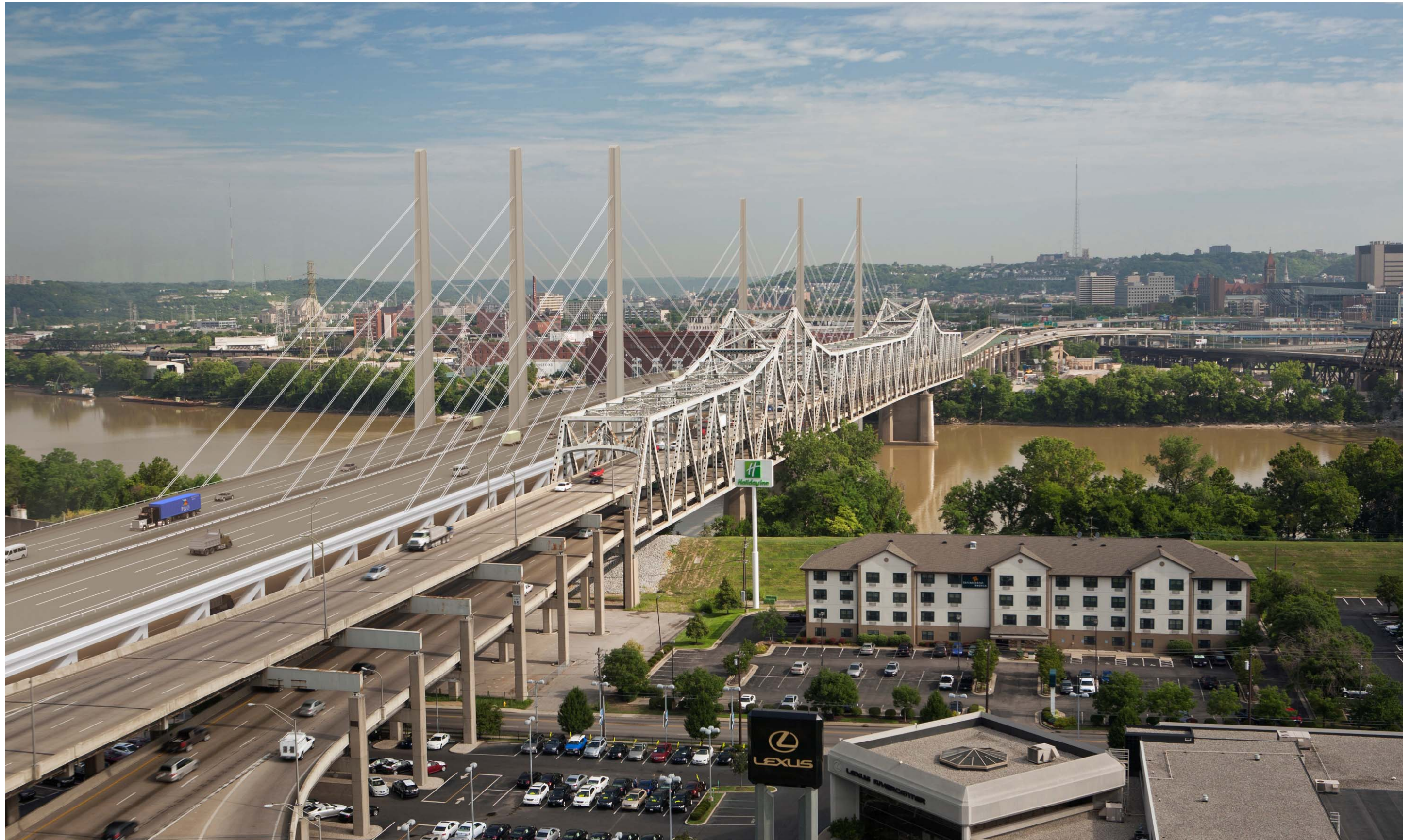
ALTERNATIVE 3 – TWO TOWER CABLE STAYED
