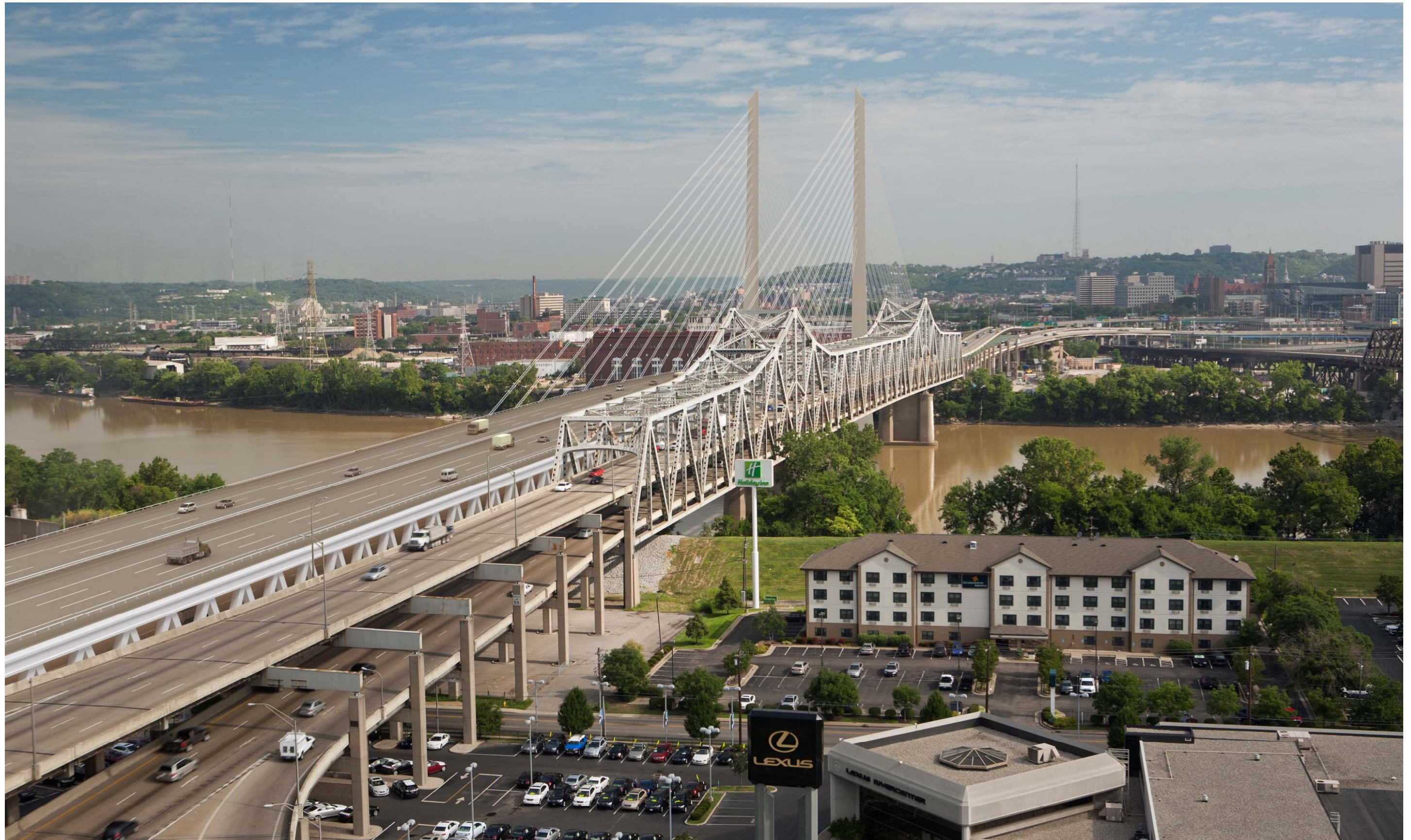
ALTERNATIVE 6 – ONE TOWER CABLE STAYED
