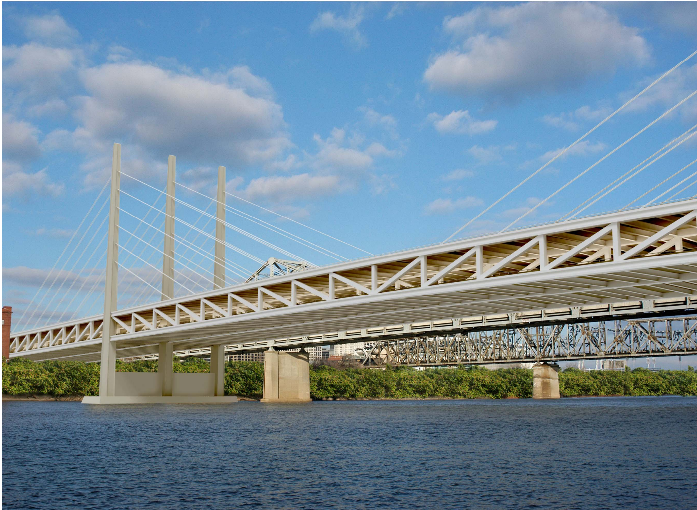
ALTERNATIVE 3 – TWO TOWER CABLE STAYED
