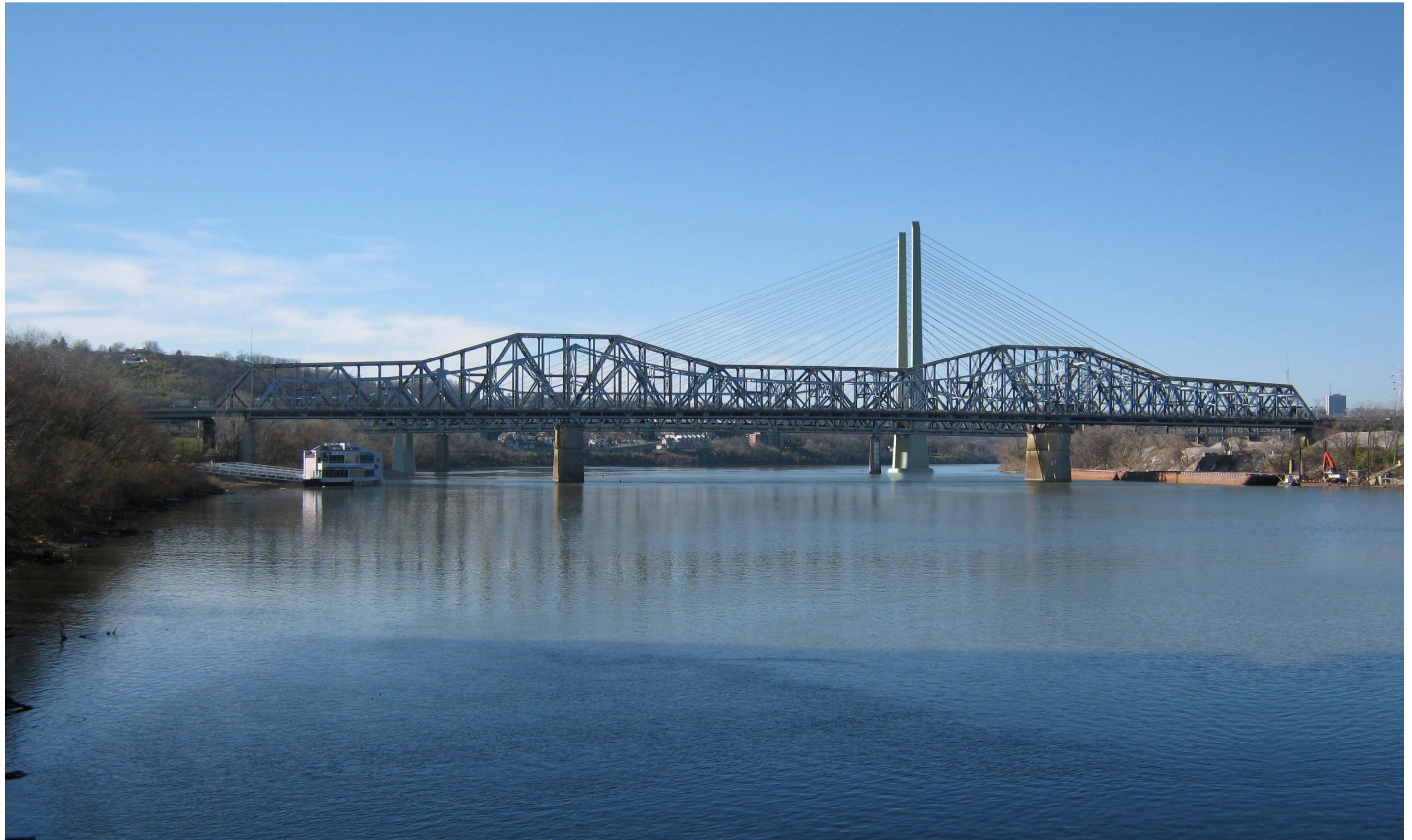
ALTERNATIVE 6 – ONE TOWER CABLE STAYED
