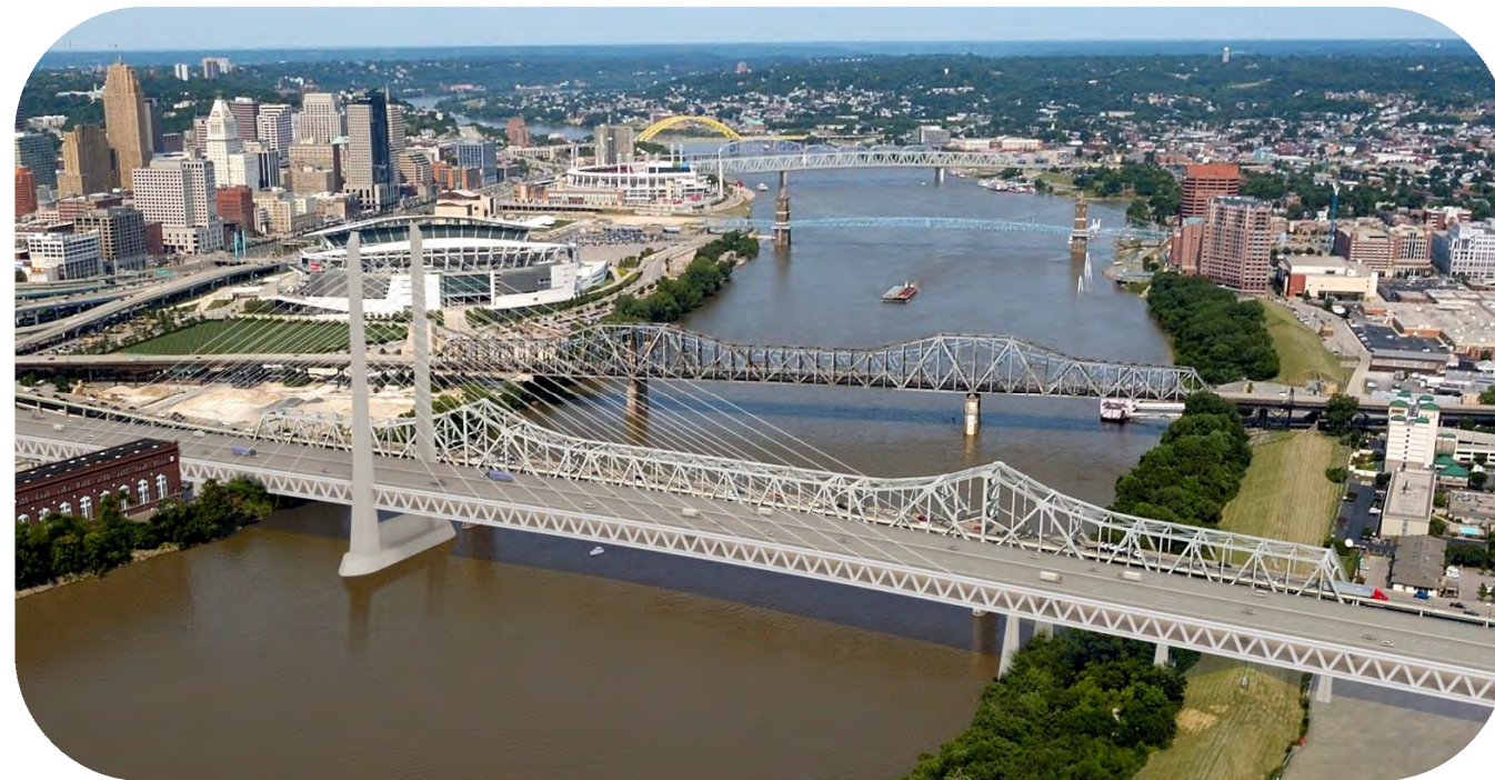
Alternative 6: One Tower Cable Stayed Bridge
