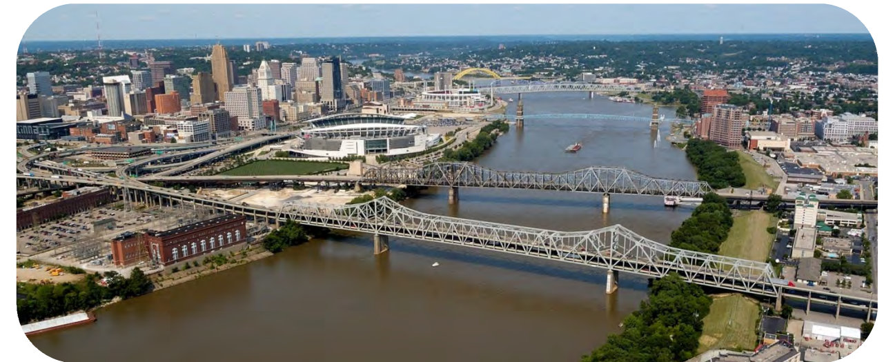
Existing Brent Spence Bridge in Forefront
