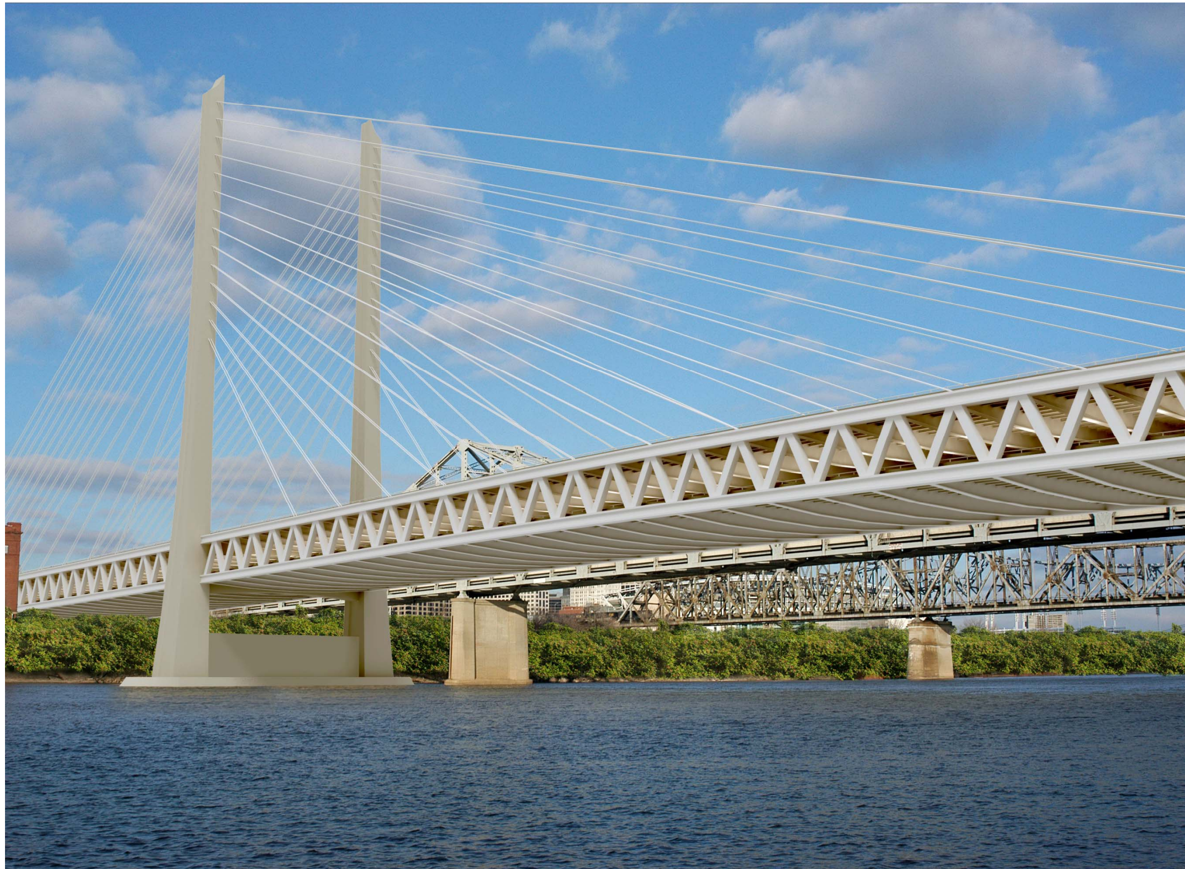
ALTERNATIVE 6 – ONE TOWER CABLE STAYED
