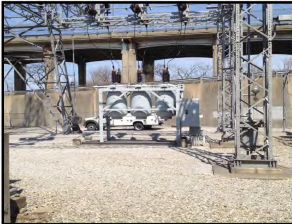
Photo #18 Circuit breakers located in substation yard.
