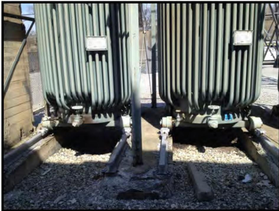
Photo #8 Transformers located in substation yard. Note staining.
