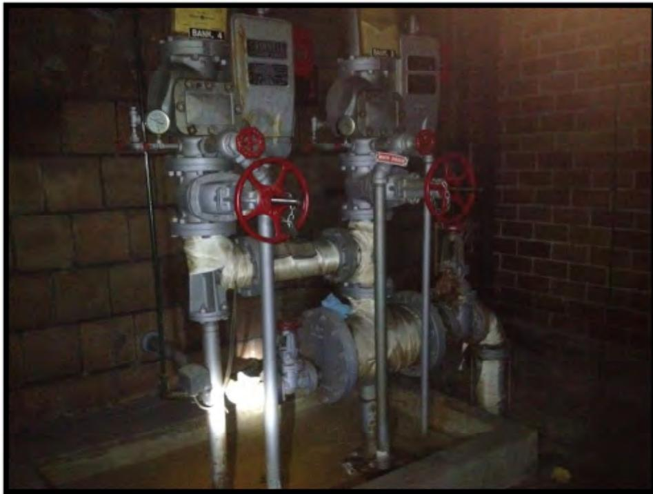
Photo #28 Emulsifier for transformer yard located on 1<sup>st</sup> floor of building.
