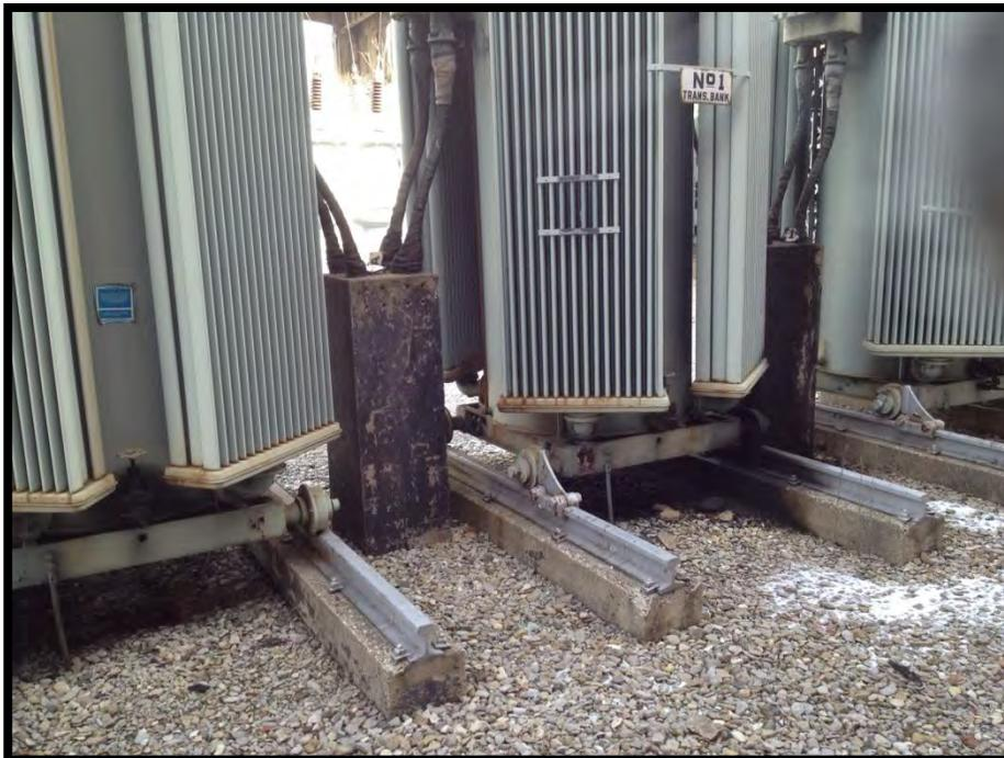
Photo #18 View of oil staining beneath transformers.
