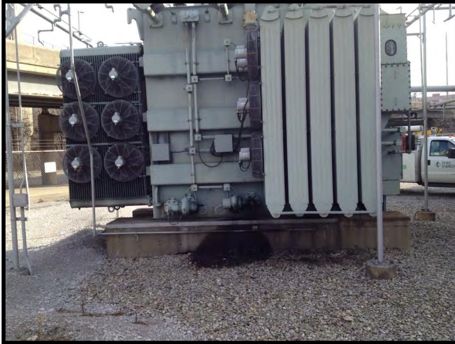
Photo #19 View of control panel and transformer, note staining.
