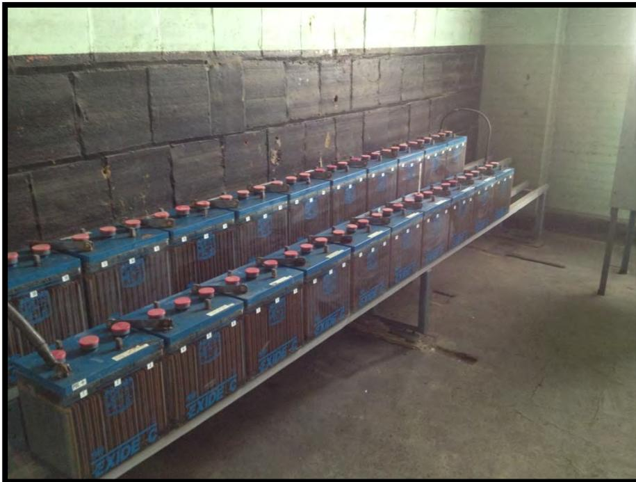
Photo #30 Backup battery storage of 2229 Spring Grove Avenue. First Floor.
