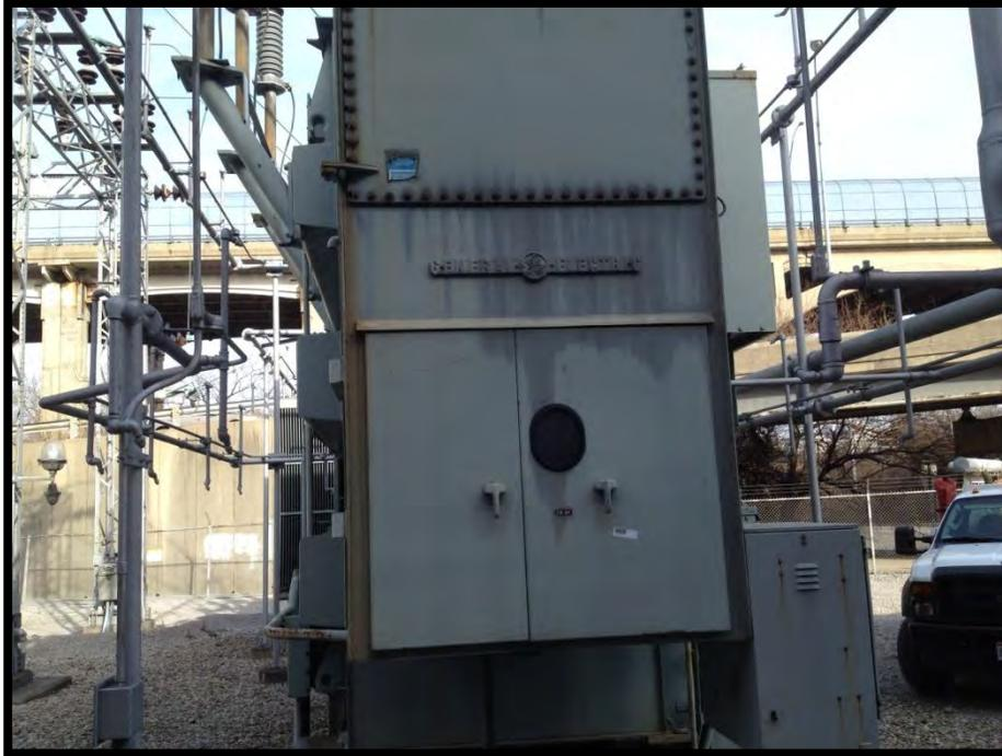
Photo #21 View of transformer, note blue “Non-PCB” label.
