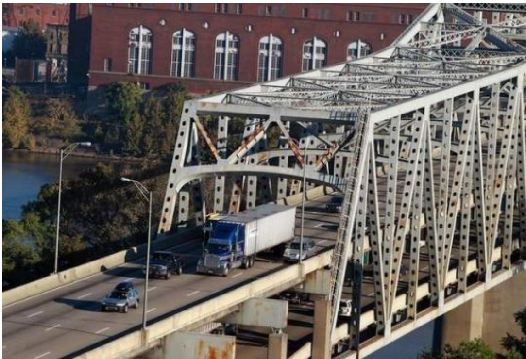
Exhibit 2-1: The Existing Double-decker Brent Spence Bridge
