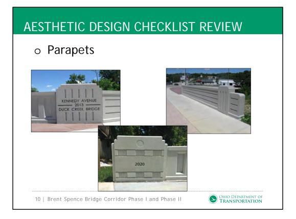
The overhead bridge parapets will also include end treatments with the bridge identification name, construction completion date and rustification design features – The city will assist in determining the final design of the parapet end treatments
